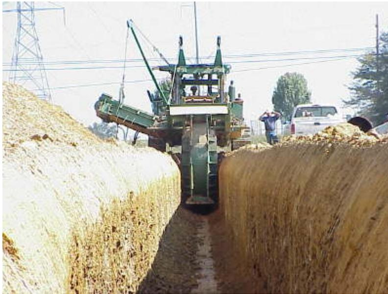
**FIGURE 3.3-9 Pipeline Ditching (Source: Photo courtesy of U.S. Pipeline, Inc. Reproduced with permission.)**
