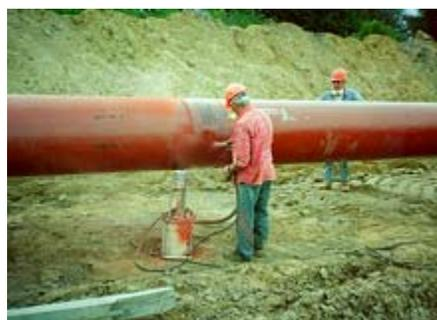
**FIGURE 3.3-12 Applying Coating to Pipeline**
