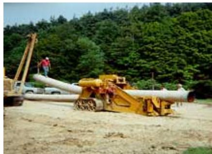
**FIGURE 3.3-11 Pipe Bending Machine**
