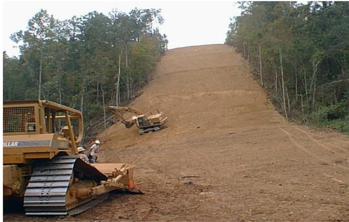
**FIGURE 3.3-15 Final Contouring of Pipeline ROW**
